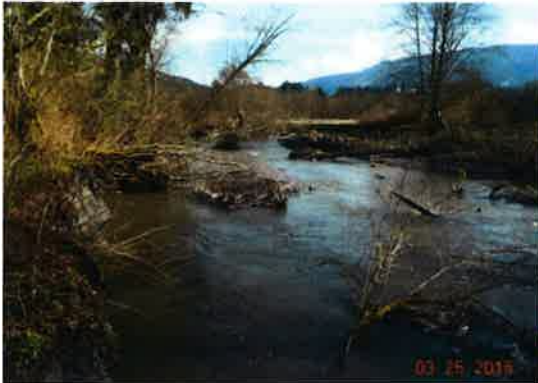
Photo 1 - View north showing active channel and cut left bank. Note erosion and recruitment of woody debris into channel.
